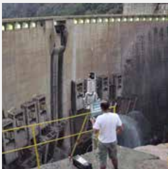
Advanced engineering technologies using laser scanning for monitoring the Cahora Bassa Dam, Mozambique, one of the largest dams in the world. © Antonio Berberan, Eliane Portela and João Boavida
