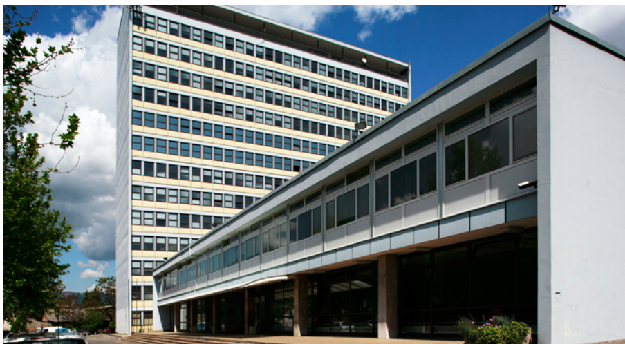
Figure A.1. UNIZGFER skyscraper building.
