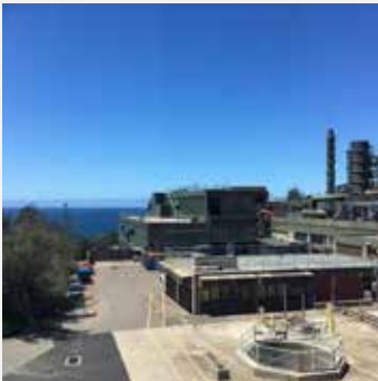
Biogas from treated sewage used to generate electricity at North Head Wastewater Treatment Plant, Sydney, Australia. © Marlene Kanga
