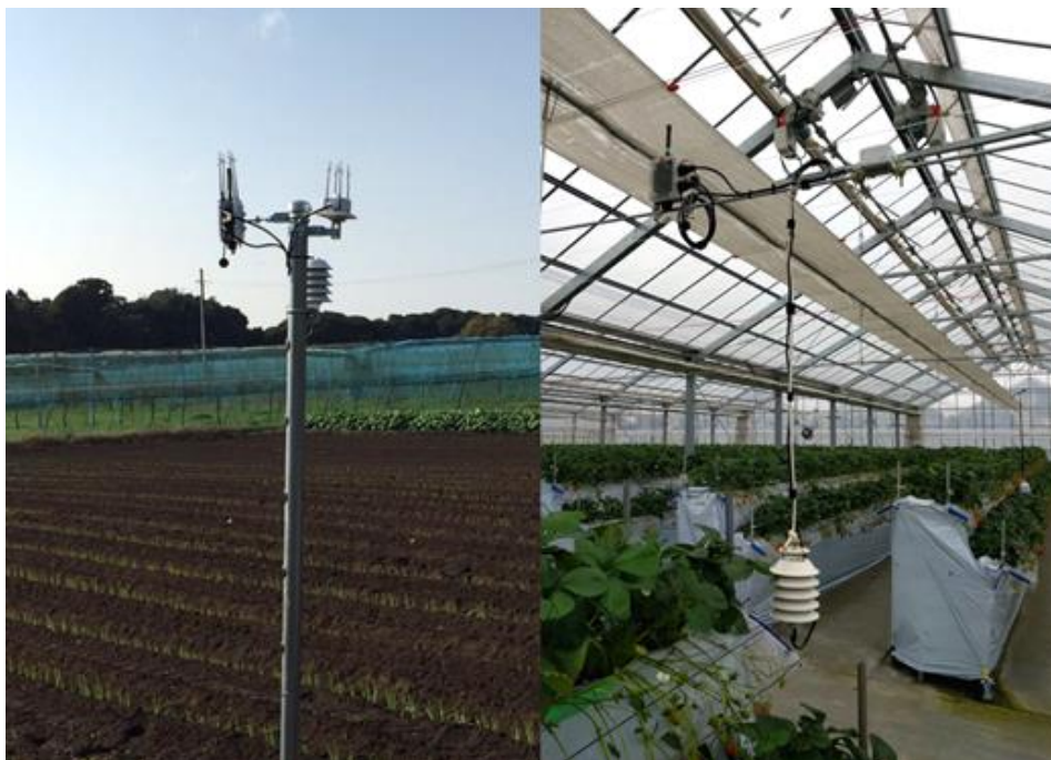
Figure 5.11. A sensor module with illuminance and ambient air temperature and humidity sensors attached, at the Chiba and Niigata test sites in Japan. Left is the outdoor installation in an onion field (Chiba) and on the right is the installation in a greenhouse used to grow strawberries (Niigata).
