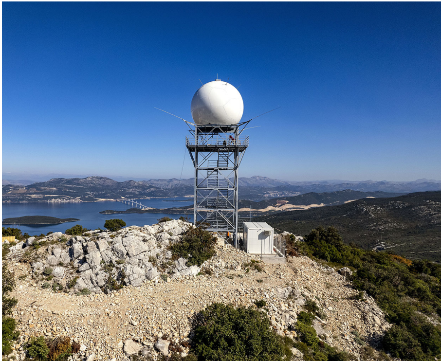
Figure 2.1: Radar on a specially designed tower located at meteorological radar center Uljenje in Croatia [6]
