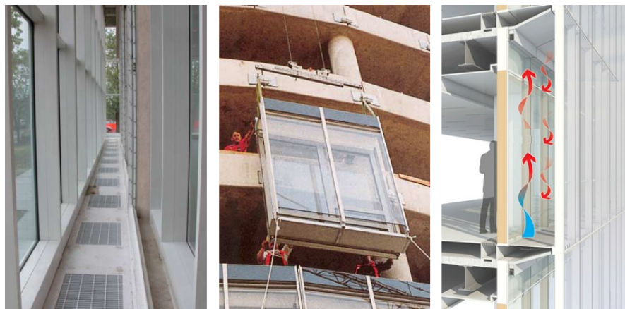
FIGURE 2.2. Examples of corridor double skin façade system a) Occidental Chemical, Niagara Falls L[32], b) Business Tower, Nuremberg L[33], c) Cutaway L[34]]
