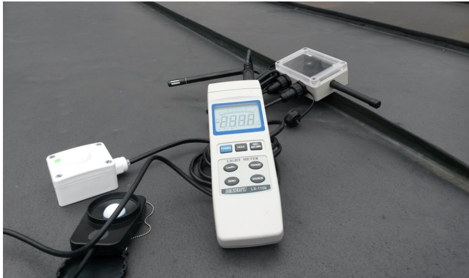
Figure 5.1. A sensor module placed on the roof during sun charging tests. Digital illuminance sensor (white box), reference light meter with the sensing element (black box) and an analog ambient temperature and humidity sensor are displayed.
